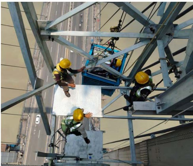
Second Hooghly Bridge rehabilitation, Kolkata
