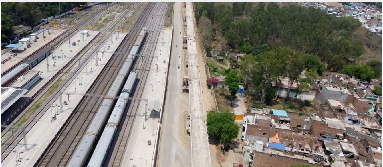
Prayagraj Rail Flyover
