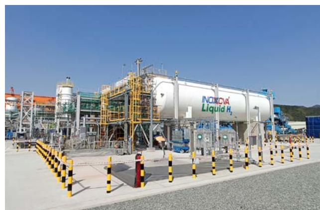
Our first installation of Liquid H2 tanks now commissioned in South Korea, which are used for mobility application.
