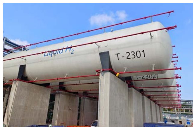
Our first installation of Liquid H2 tanks now commissioned in South Korea, which are used for mobility application.
