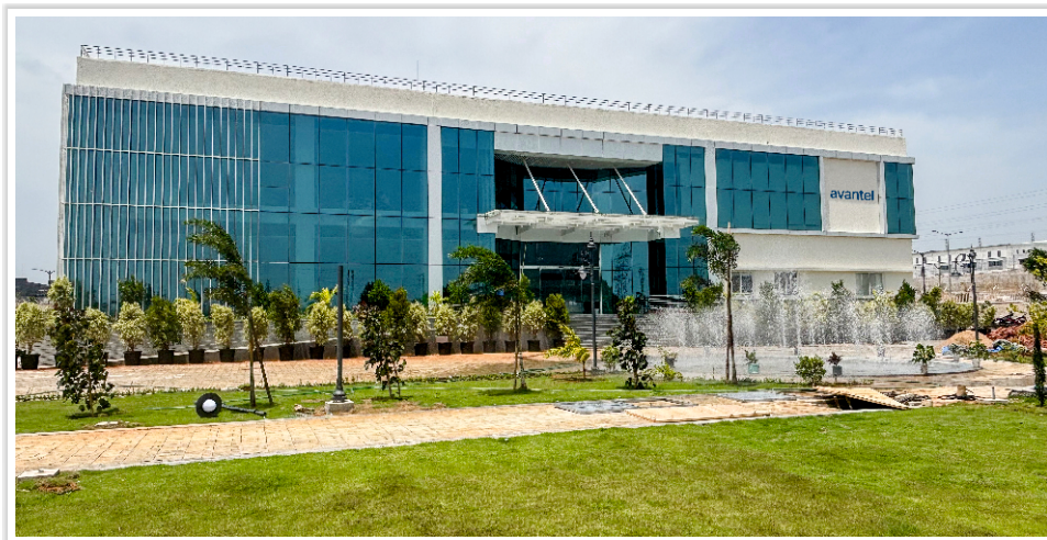
Photo of Avantel, E-City Facility, Hyderabad
