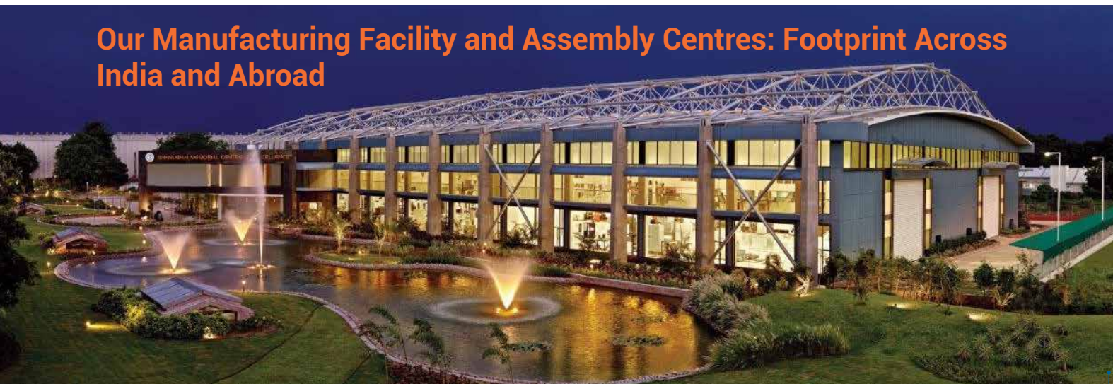
Outside view of BMCE Plant
