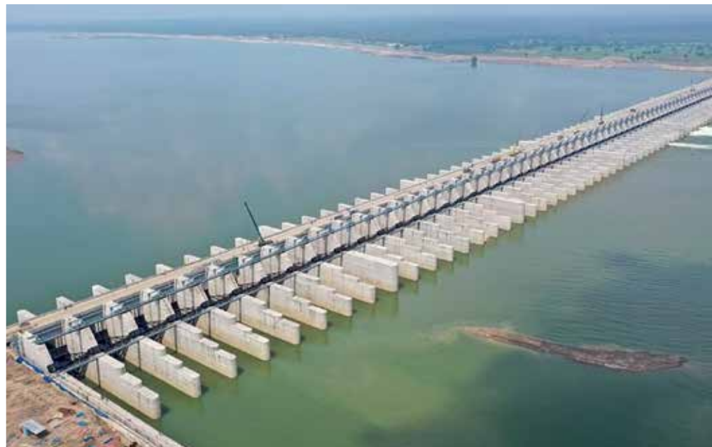
Bhanupali-Bilaspur-Beri Railway Gauge Link Himachal Pradesh
