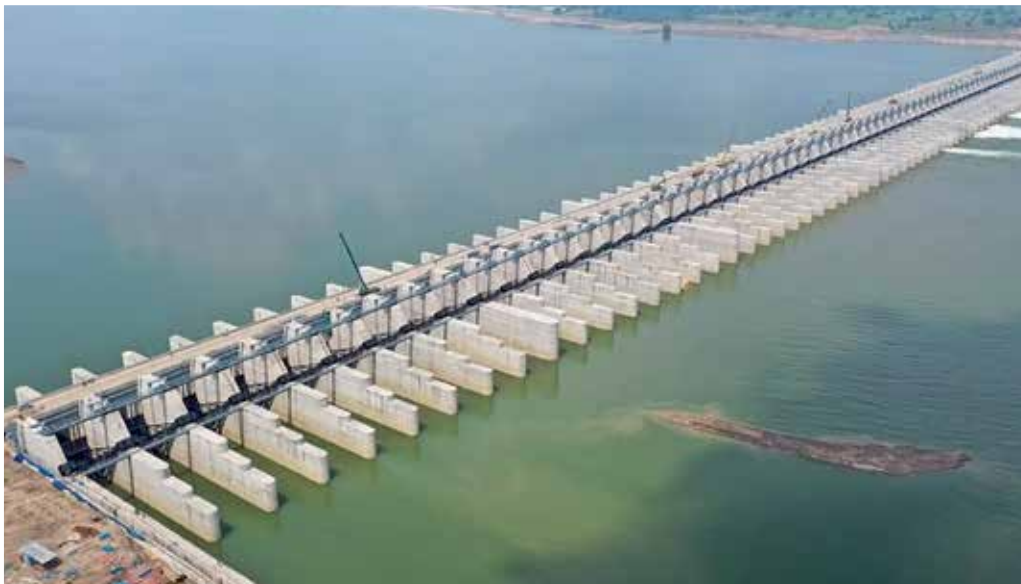
Lift Irrigation Project Kaleshwaram Bhupalpally, Telangana
