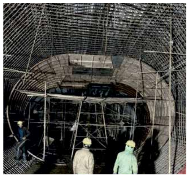
Shongthong Karchham Hydro Electric Project, Himachal Pradesh
