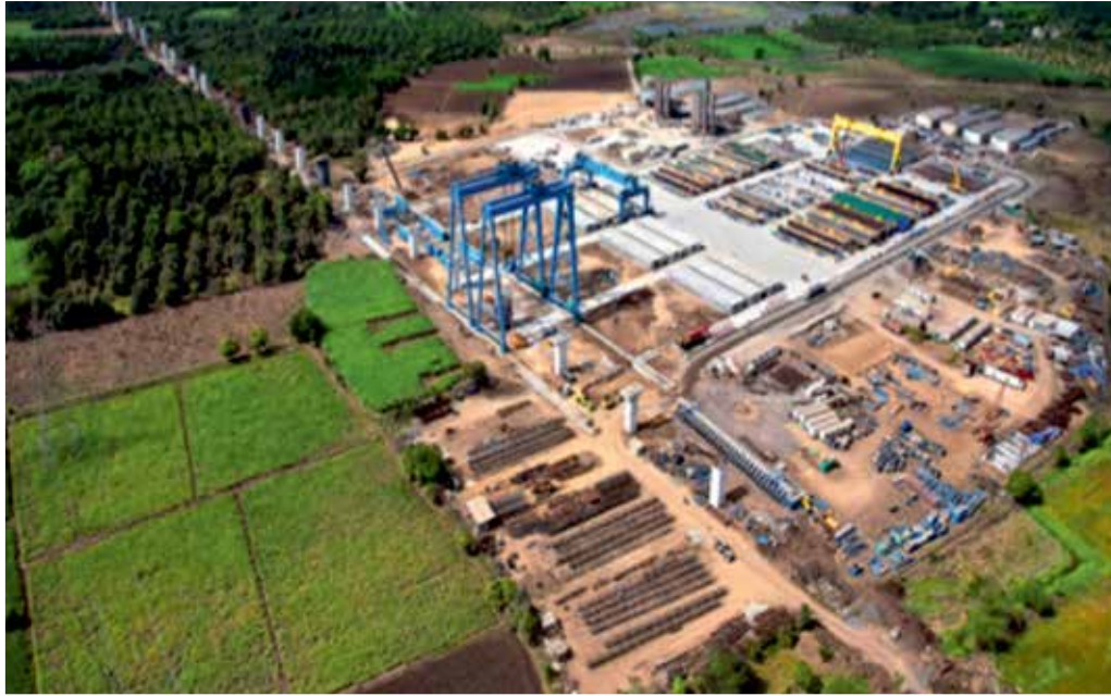
Mumbai-Ahmedabad High Speed Rail Project
