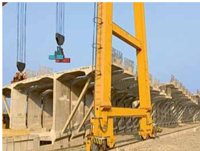
Assam-Meghalaya Dhubri Bridge
