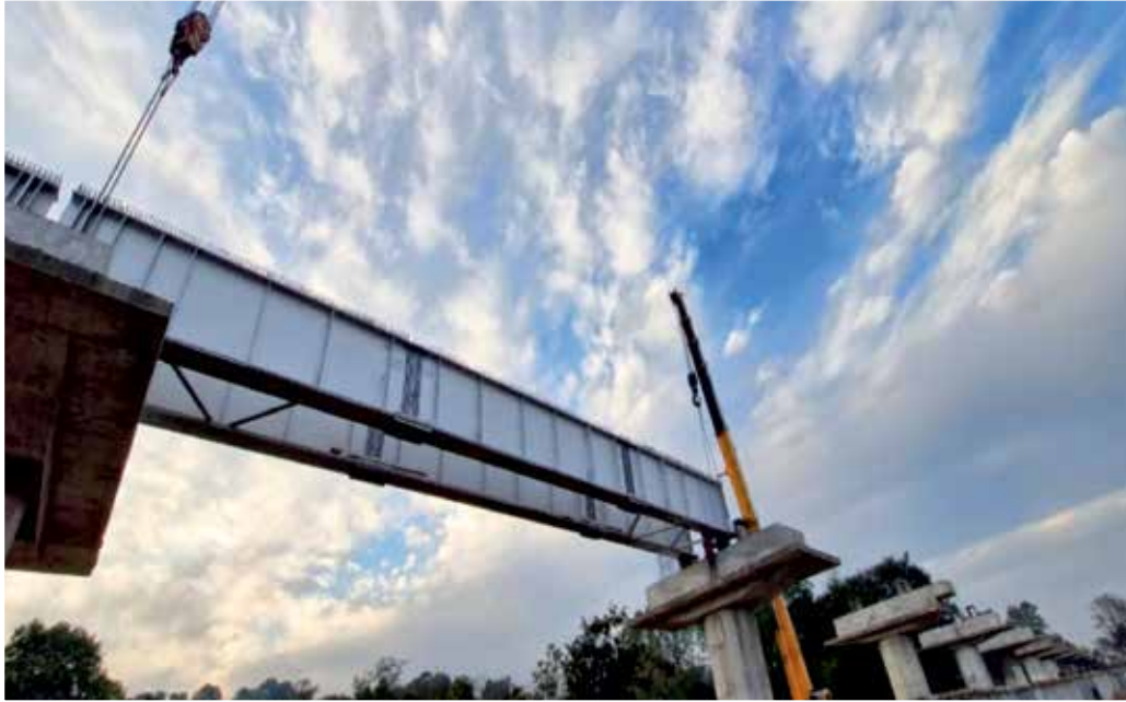
Nangal Dam-Talwara New BG Rail Link Daulatpur Chowk (Himachal Pradesh) to Kartoli (Punjab) Block Section
