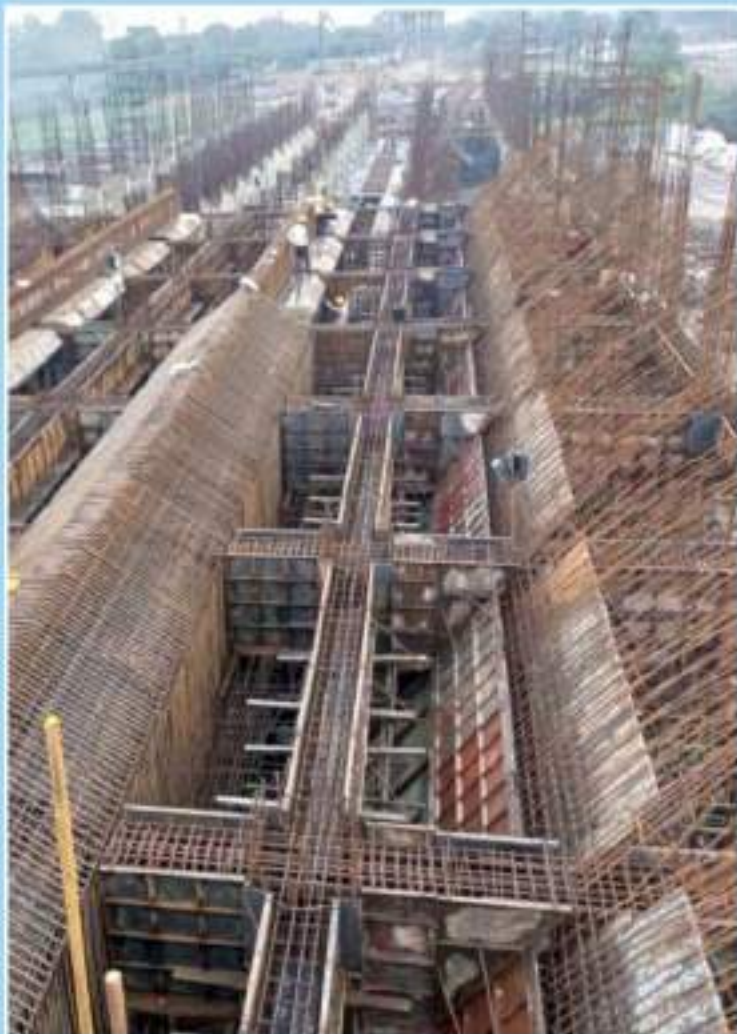
Construction of 20000 tonne capacity over ground coal storage bunker for 9.50 MTPA NCL BINA KAKRI Project is under progress
